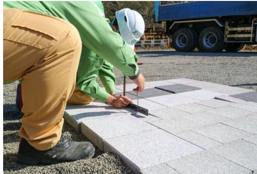
Step Measurement by Calipers
