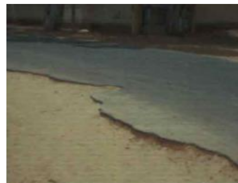
Fig 8 : Shore lace or spalling
